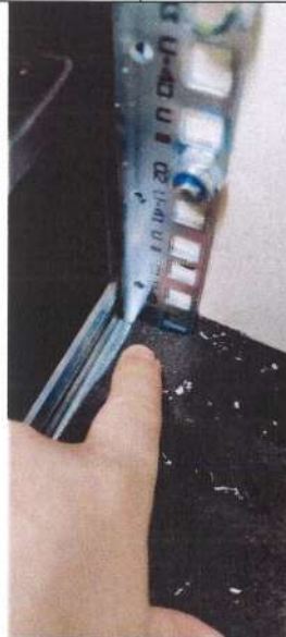
42U (W=750X,D=1130XH=2110) Cabinet internal frame
