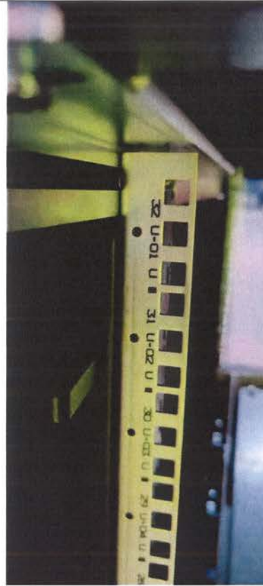
32 U (W=750X,D=1130x H=1666) Cabinet internal frame
